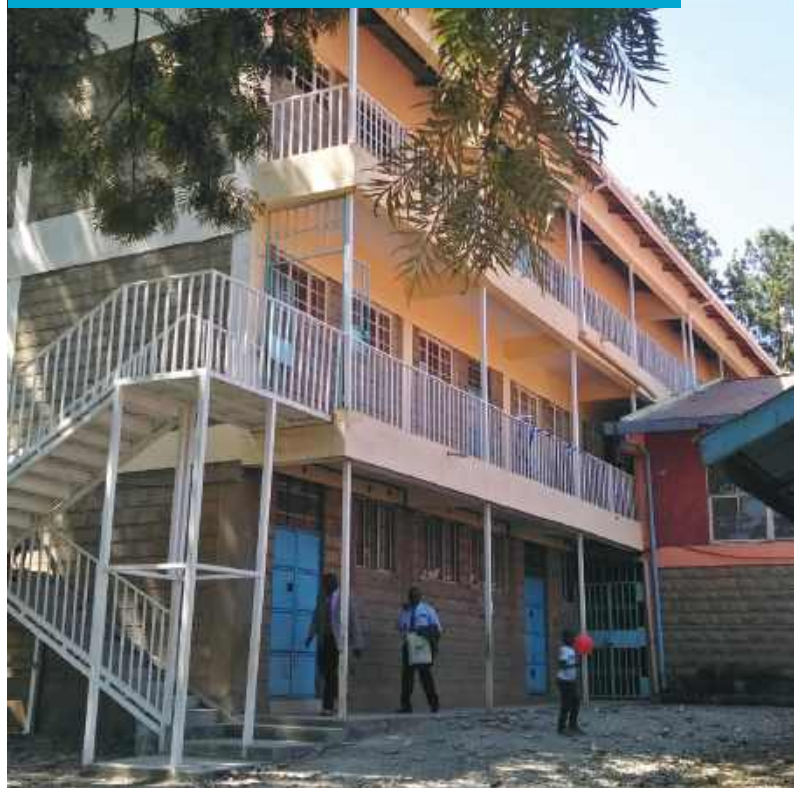
Front (side) elevation of the completed facility during the official opening day at PCEA Emmanuel church - Kibra
